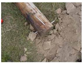
Figure 2 Brace Pins
